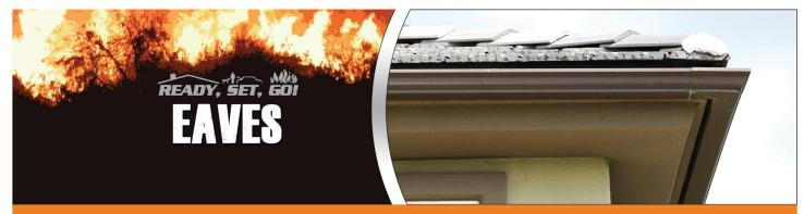
Eaves are the underneath part of the roof that extends beyond the home's outer wall to the roof's edge.
