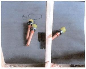
heads can be installed ONLY after all CPVC pipe and fittings are solvent cemented to the piping system and allowed to cure for a minimum of thirty (30) minutes."
